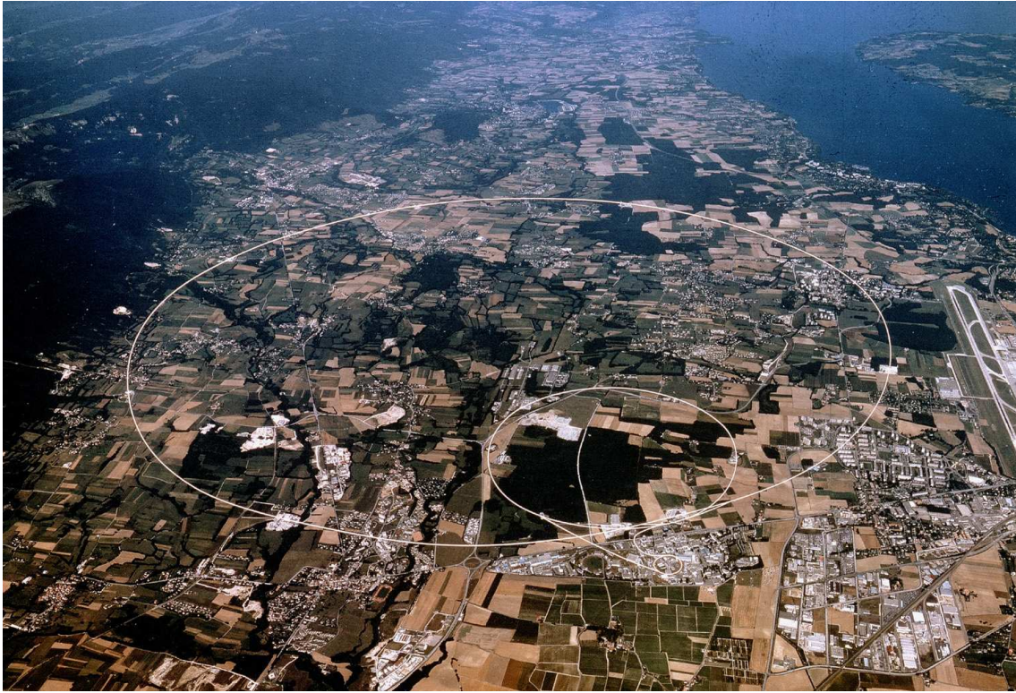
Figure 3.1: An aerial view of the LEP tunnel which is re-used for the LHC accelerator [15].
