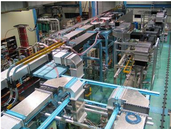
Figure 1: Overall system of PEFP 20 MeV accelerator.
