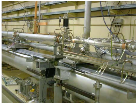
Figure 5: The first prototype 1m-long accelerating section installed in the beam line of the KEKB/PF linac.
