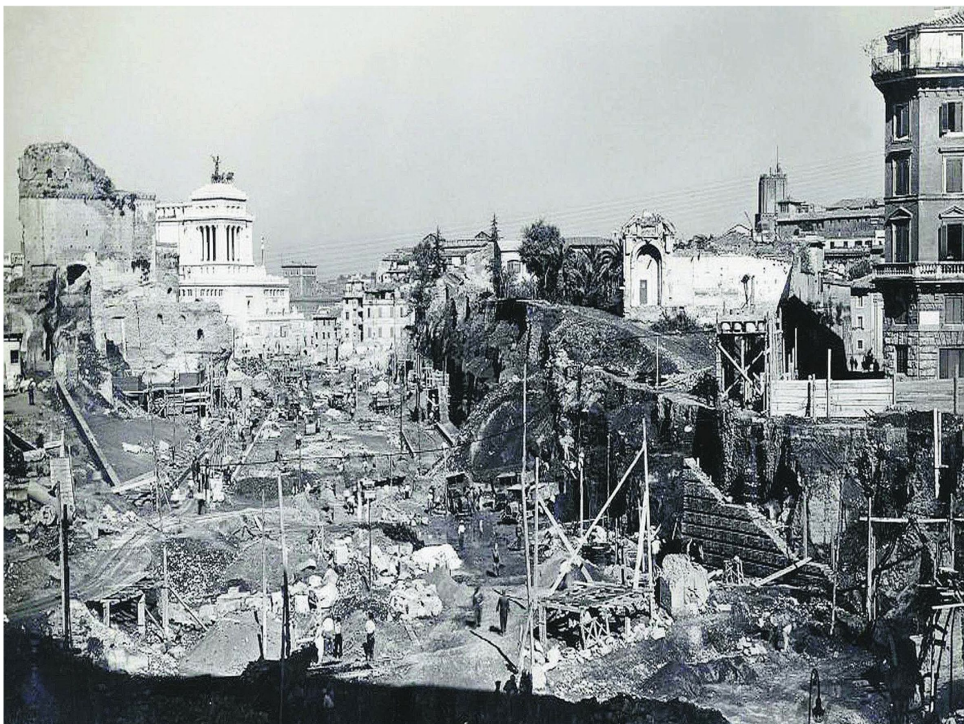
Figure 4. Picture published in media in October 1932, depicting the excavation works for the opening of the VFI and the dismantling of the Velia hill (credit Archive X division Municipality of Rome).
