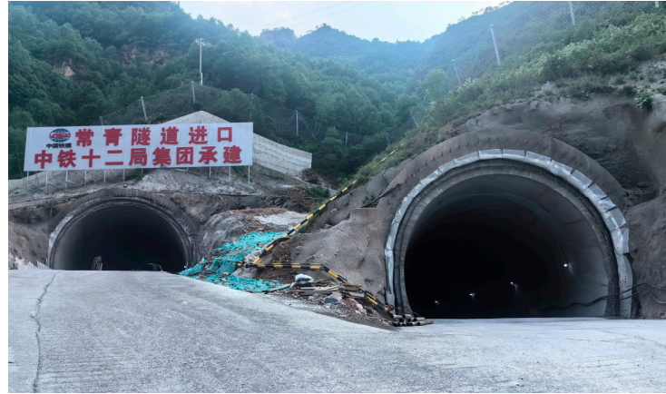
Figure 10. A section of closed tunnel in Xiongqin (Xiongan to Qinzhou).
