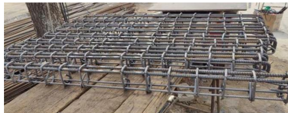
Figure 3. Steel skeletons of the beams.
