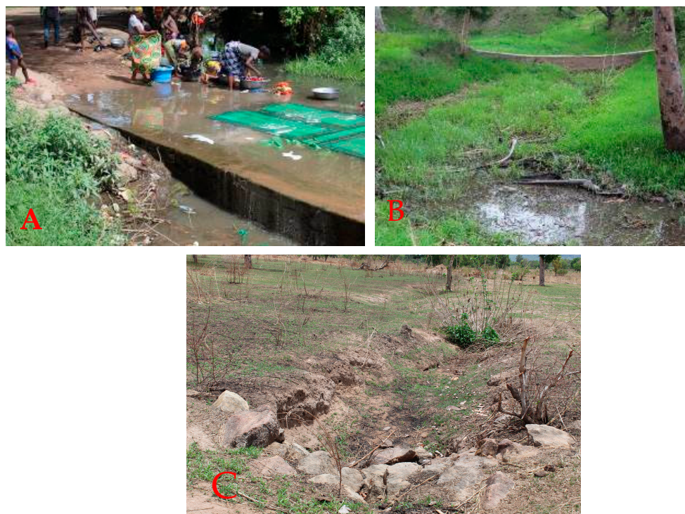
Figure 6. Masonry (A,B) in Ndock and stone wedged “biefs” (C) in Sabongari. (Source: Tchuenga, March 2022).
