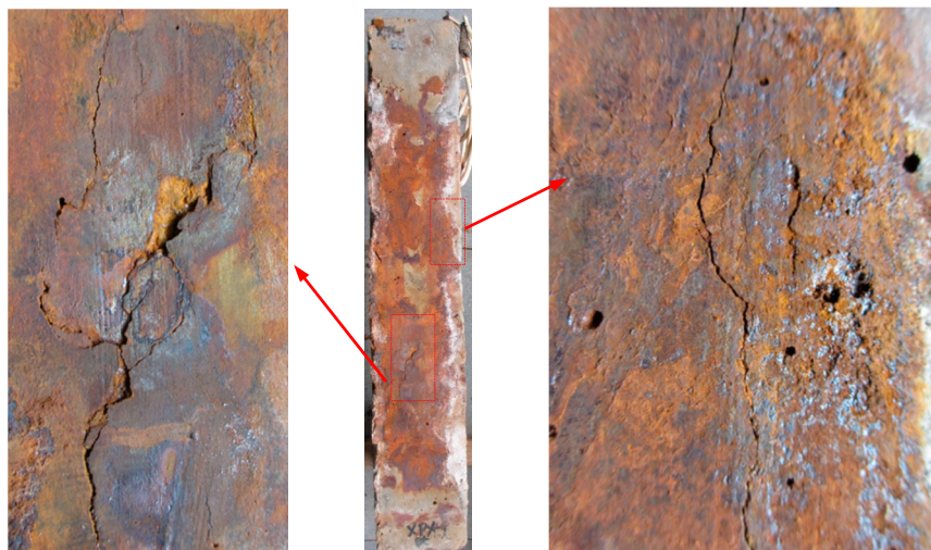
Figure 12. Cracks due to volumetric increase by rust formation on the surfaces of the RC column specimens.
