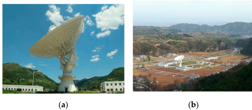
Figure 2. The (a) and (b) show the 40 m dish antenna and its surrounding environment respectively.
