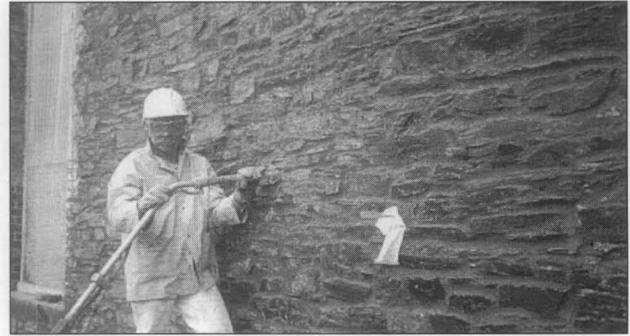
17. The internal grout injection of rubble walls can improve seismic capacity. Care must be taken in formulating the mortar grout and repairing the area where injection occurs. Photo: Architectural Resources Group, San Francisco.
