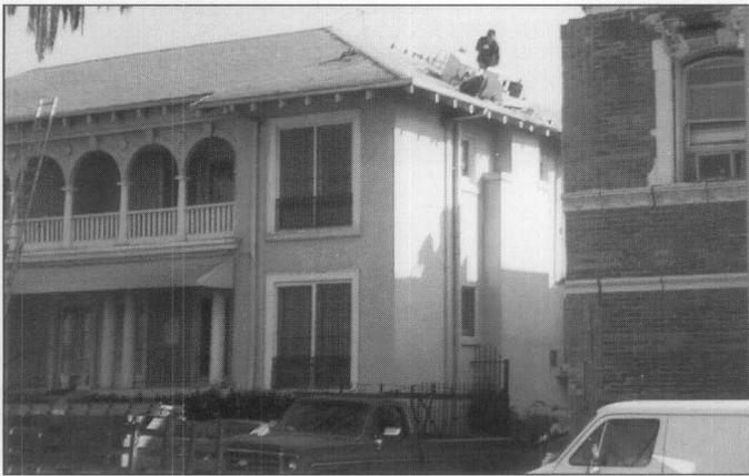
4. The compact size and good condition of the masonry building on the left withstood the earthquake except for the loss of the unsupported chimney at the roof line. The brick building on the right appears to have sustained more damage. Photo: Steade Craig.
