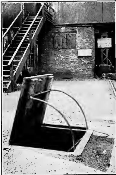
PLATE 15.—PROTECTIVE DEVICE FOR TRAP DOORS
