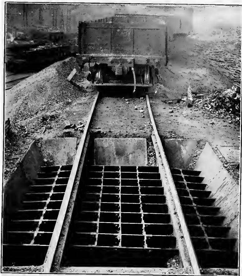
PLATE 18.—GRILL WORK PROTECTION FOR BINS AND HOPPERS or ore, into the bin underneath if not gotten out promptly
