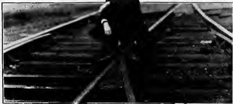
PLATE 17.—GUARD FOR FROGS MADE OF STEEL PLATE
