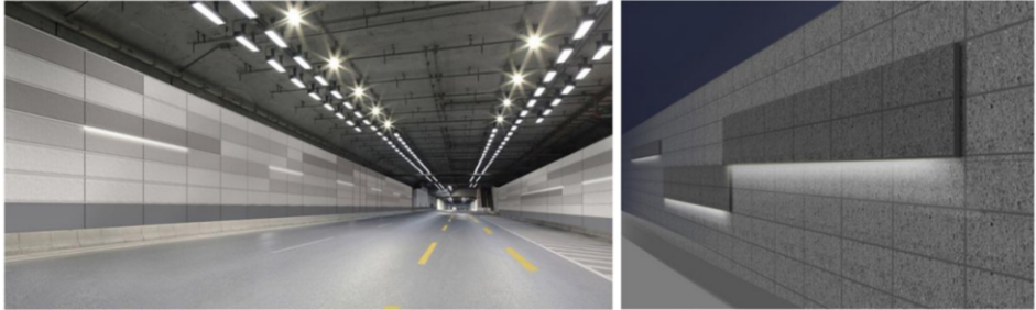
Figure.12 Beijing East Sixth Ring Road Tunnel.
