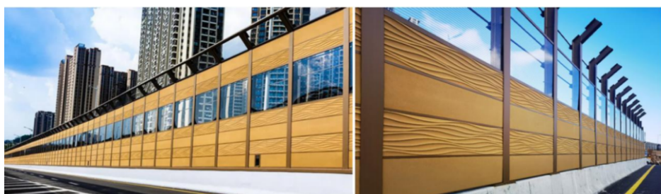
Figure 7. Noise barrier of Shenzhen Pingyan Expressway.
