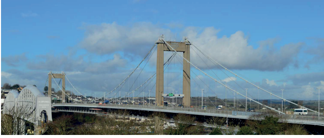
Figure 2. Tamar Suspension Bridge (UK): view from the Devon bank.
