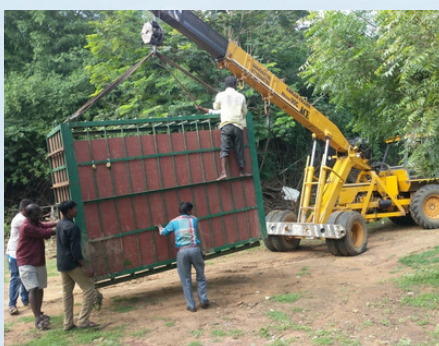
Unloading of crate with the help of crane
